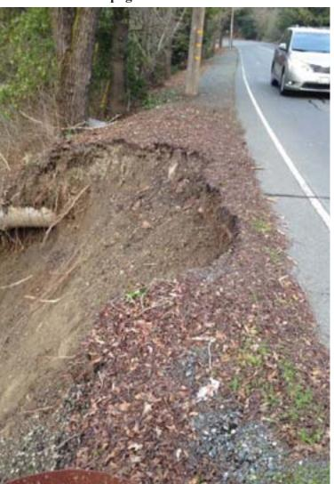
St. Mary's Road at the point of slide – exposed pipe visible. "The gas is located near the failed shoulder of the road and that was my biggest immediate concern."
